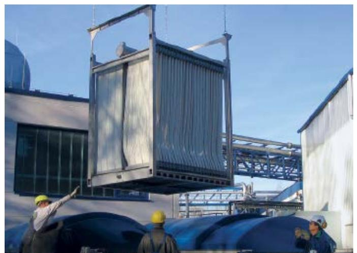
Abb. 3: Membranfiltrationskassette ZeeWeed 500 D
