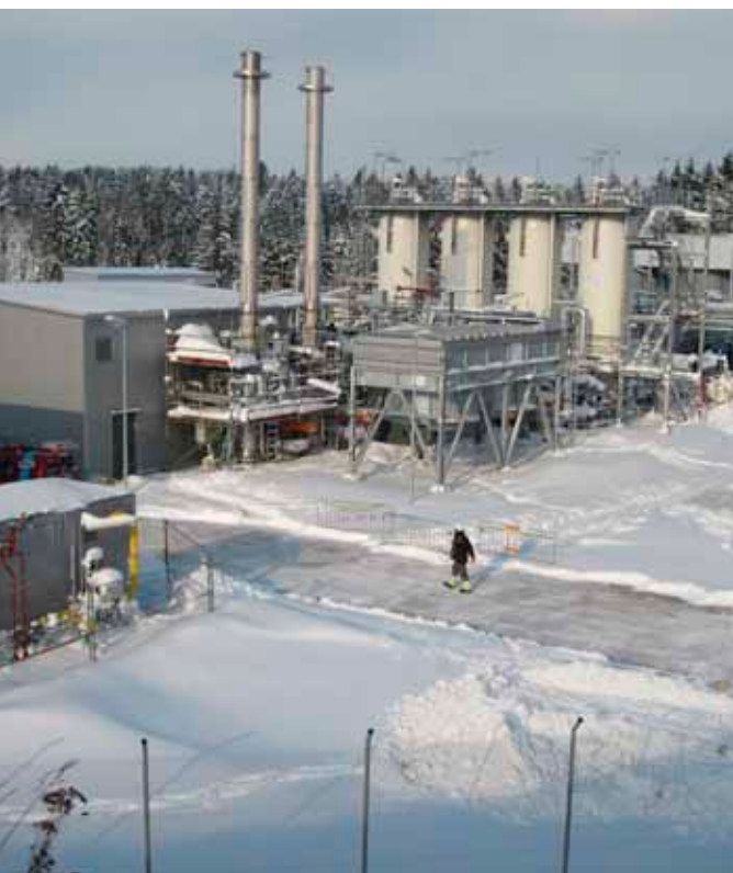
Montage in Zagling
