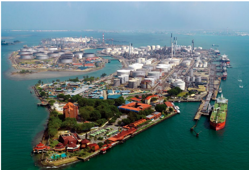
Growing demand in Asian economies led Western chemical manufacturers to invest heavily in the region. The photo shows the fully integrated Shell Eastern Petrochemicals Complex in Singapore.
