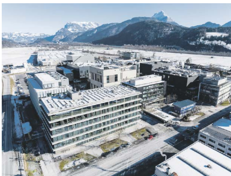
Novartis plant in Tyrol, Austria
