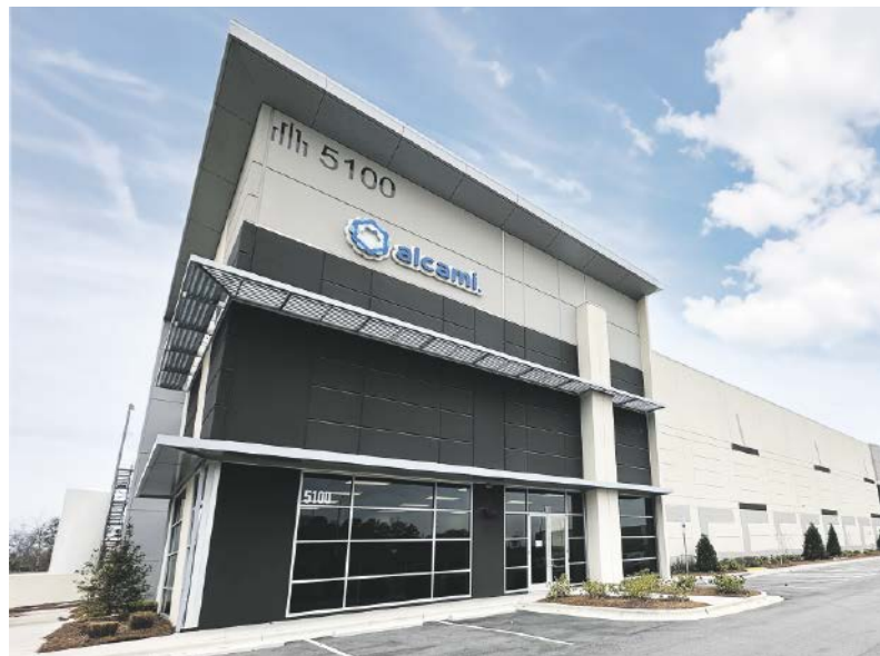
Alcami's advanced pharma storage and services facility in Garner, NC, USA
