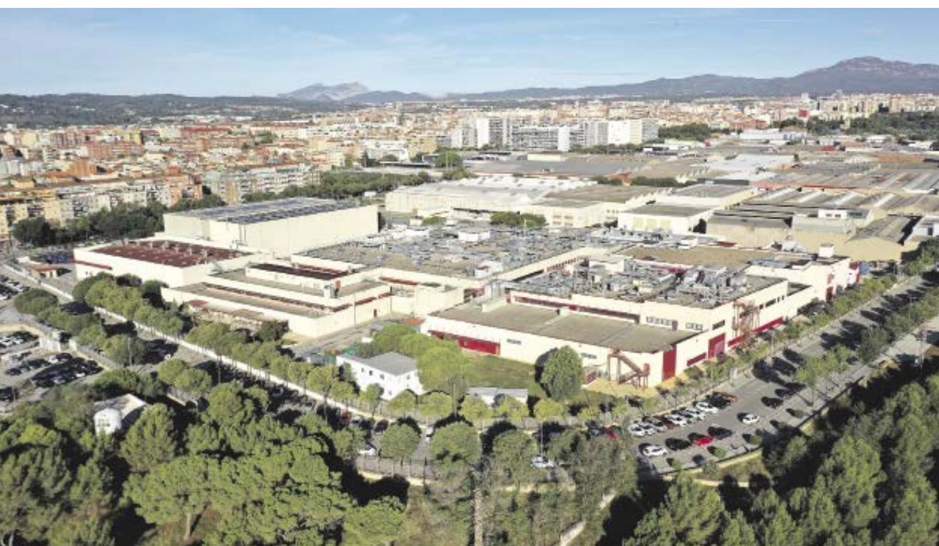
Aerial view of Siegfried's site in Barberà del Vallès, Spain
