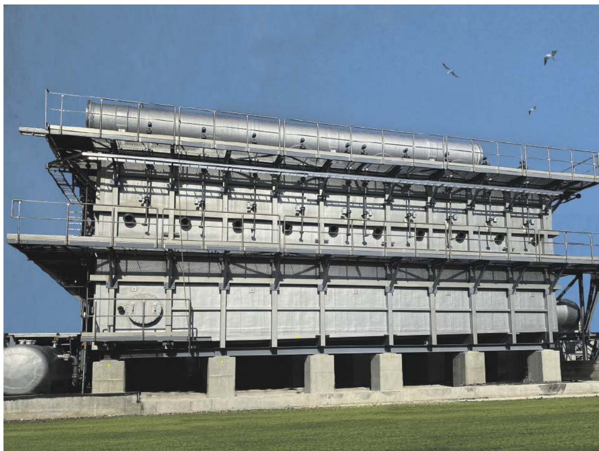
Exterior view of KVT's Oxysulf reactor.
