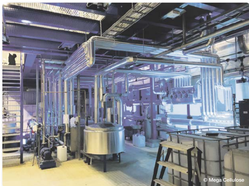
Mega Cellulose plans to build and operate a modular multi-product synthesis plant for chemical modification of natural polymers.
