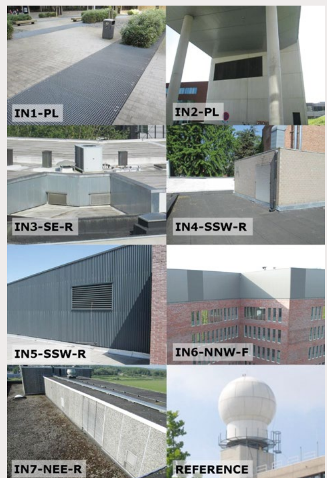
Fig. 1: Air intake configurations
