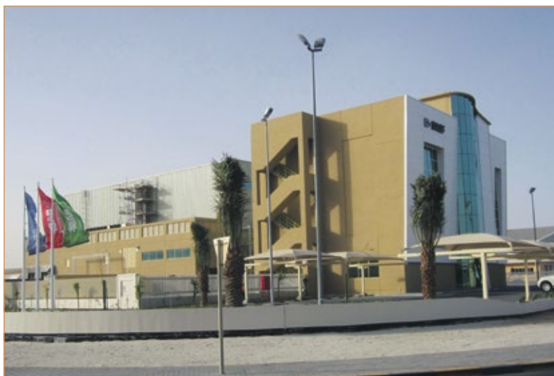
BASF's new plastics additives facility in Bahrain.
