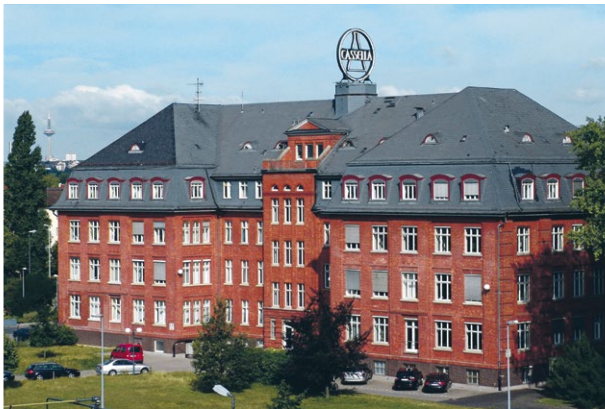
This historical building in Cassella Industrial Park in Frankfurt houses Allessa's head office and the offices of its managing directors.
