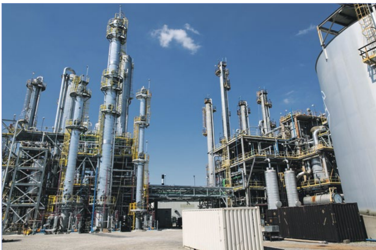
Greenfield Specialty Alcohols' Chatham facility, located in southwestern Ontario, is in the process of completing a $40-million investment to upgrade the corn-based industrial alcohol production, bringing to $300 million the total investment in the Chatham plant since it opened in 1998.
