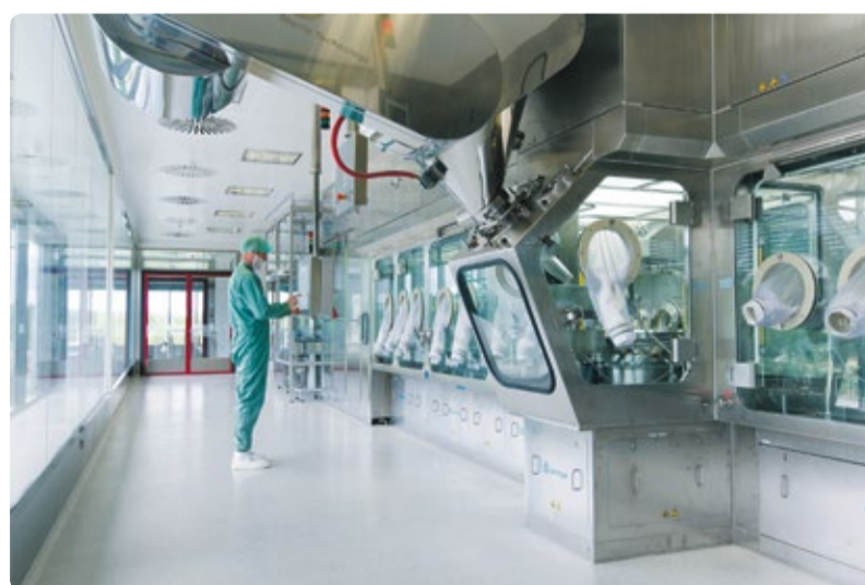
Category winner for facility integration: IDT Biologika for their multipurpose biologics and vaccines production facility (isolator vaccine filling unit) at Dessau, Germany
