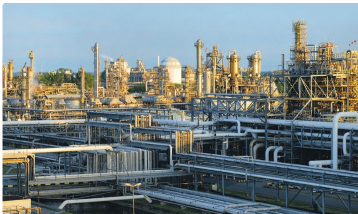
The Stade, Lower Saxony, plant of Dow Water & Process Solutions at the Elbe River between Hamburg and the North Sea.
