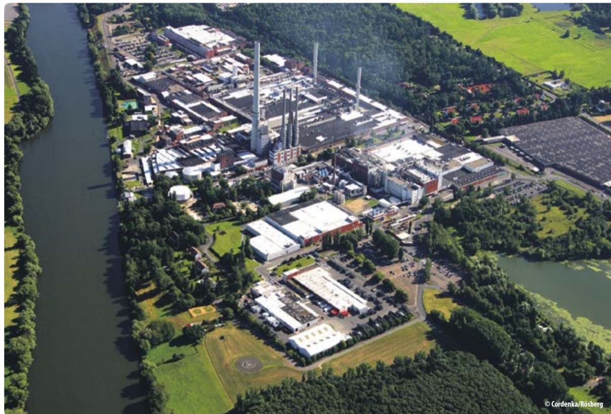
The Cordenka plant in Obernburg that has been modernized comprehensively.
