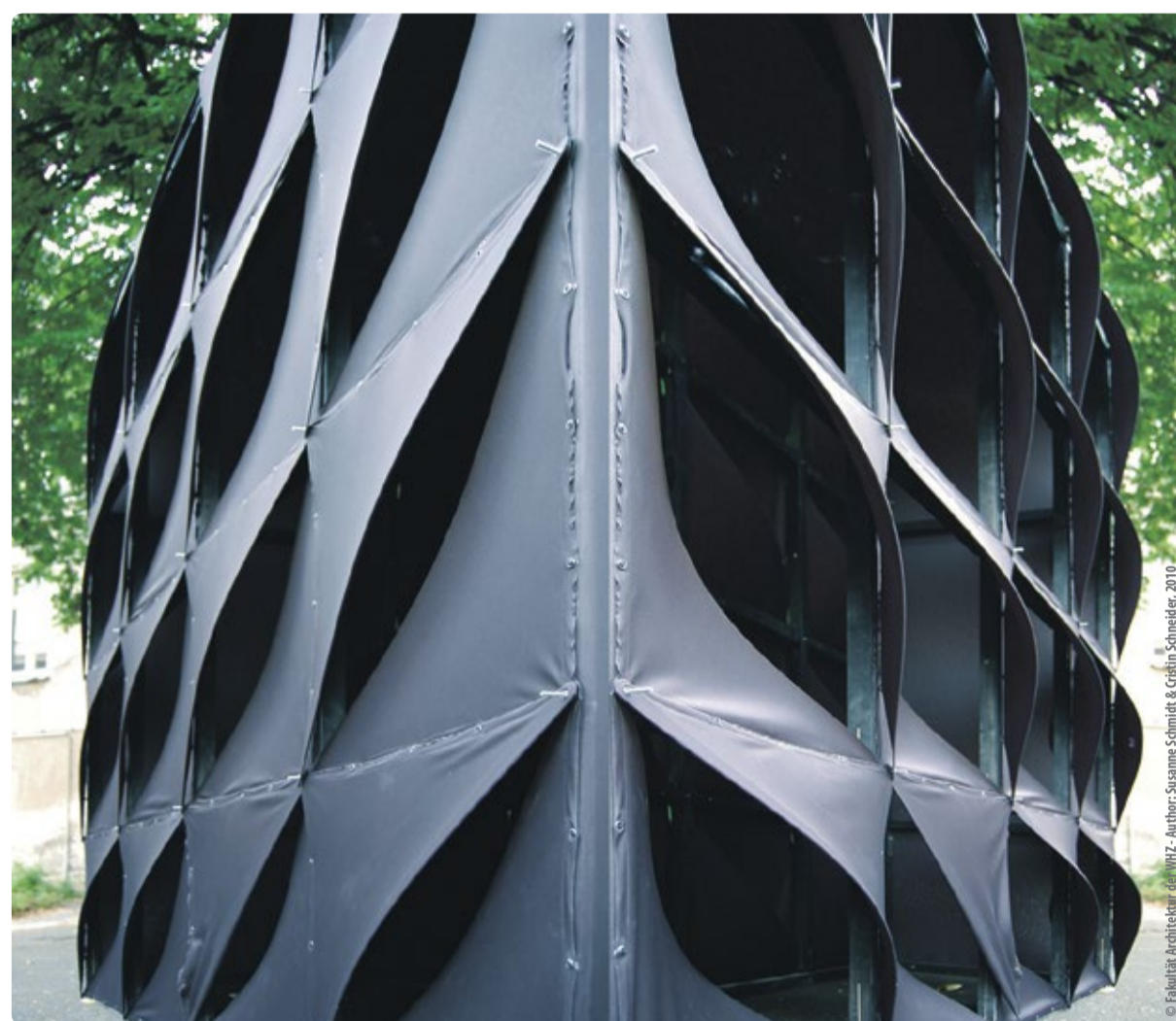
Fig.2: "Kiemenbox": the German word "Kiemen" means "gills of a fish". The slit within the facade membrane opens and closes gill-like.
