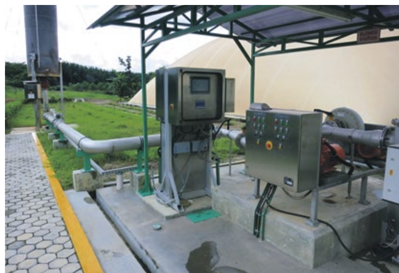
The INCA gas analysis system measures the composition of natural gas – here in a biogas plant in Indonesia.
