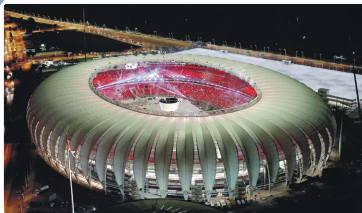
The eye-catching architecture of several venues of the 2014 FIFA World Cup has been made possible by fluoropolymers. The roofing of the Estádio Beira-Rio in Porto Alegre is made of sheets of fiberglass membranes in the shape of palm leaves that are coated with PTFE.
