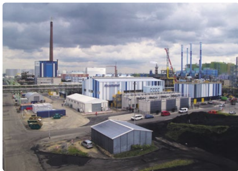
In May, AkzoNobel inaugurated its new chlorine membrane electrolysis plant in the Industrial Park Höchst, Germany (photo on the left). The state-of-the-art plant (rendering on the right) is the result of a major conversion and expansion project begun in 2011 and involving a €140 million investment. The facility has been converted from mercury cells to the latest-generation membrane technology. Capacity has been increased by 50% whilst at the same time reducing the plant's overall ecological footprint by some 20%. Radical efficiency improvements reduce energy consumption by 30% per ton of product. The facility is one of three chlorine plants operated by AkzoNobel in Germany, the other two being located in Bitterfeld and Ibbenbüren (c.f. the news below).
