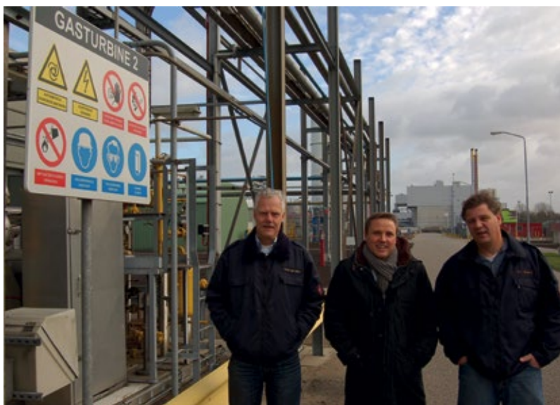
The managers of the steam saving project (from left to right): Peter van Uden, Hugo van Kempen, Erik van Kempen
