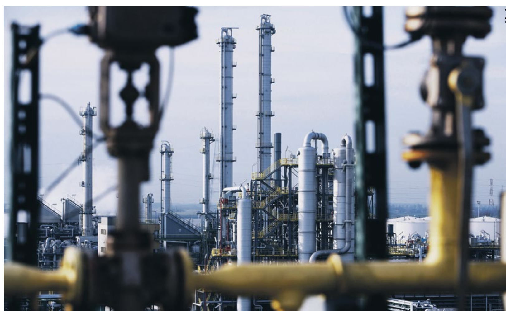
The planning of tailored chemical production plants generally still takes several years.
