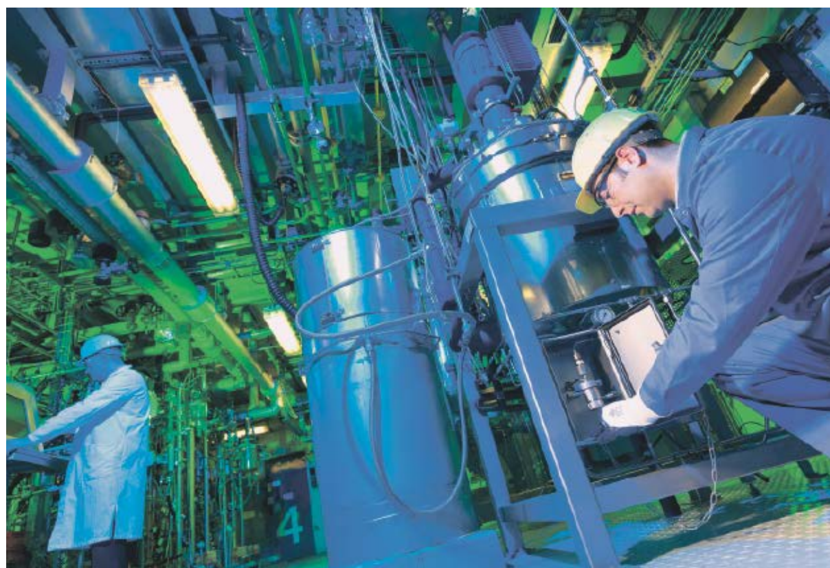
Pilot plant for production of the CO 2 -based polyols.
