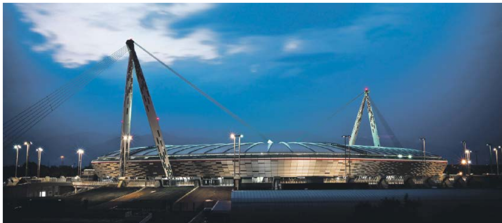
Light gray colored PVC fabric is used for the stadium cover of the new Juventus Arena in Turin, Italy.
