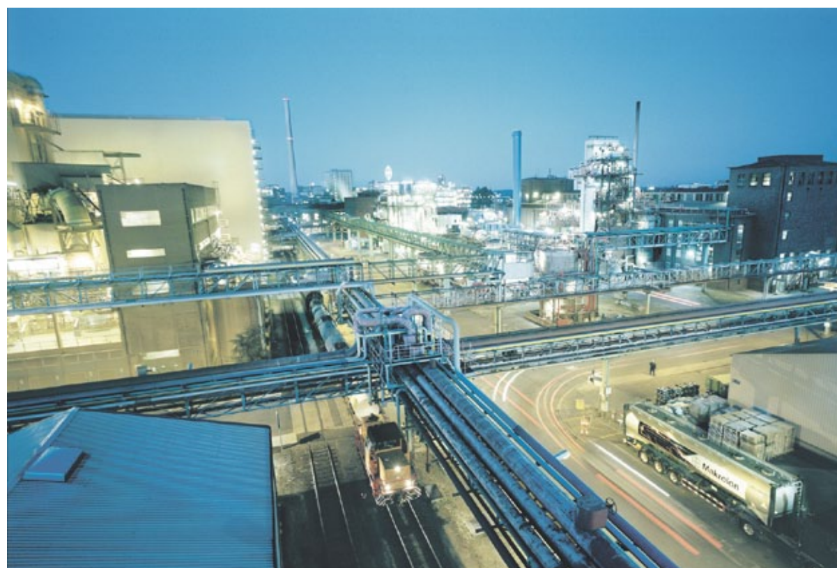
Fig. 1: Chemical site operator Currenta has invested around €1 billion in the three ChemPark sites in Leverkusen, Dormagen and Krefeld-Uerdingen. Every euro spent there draws an investment of more than three euros from ChemPark companies.
