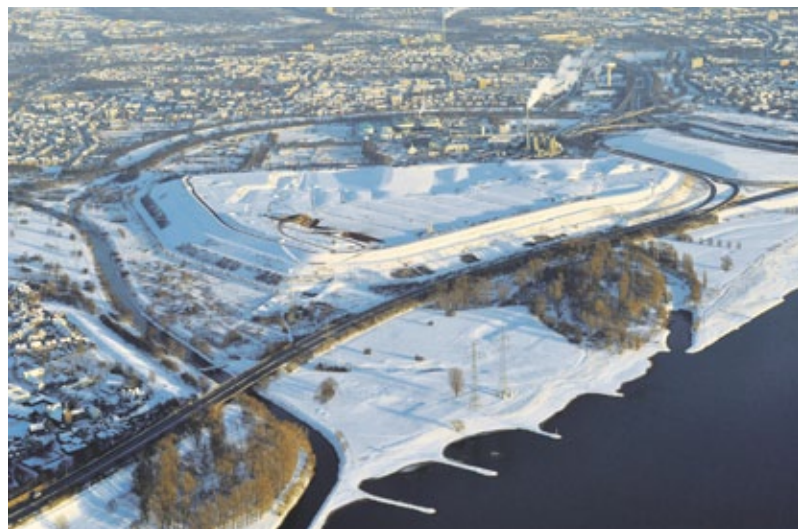
Fig. 2: The environmental experts at the Leverkusen-Bürrig Waste Management and Recycling Center are even prepared for snow and freezing temperatures. Wastewater and wastes generated by production are safely treated, thermally recycled or landfilled around the clock in both summer and winter.
