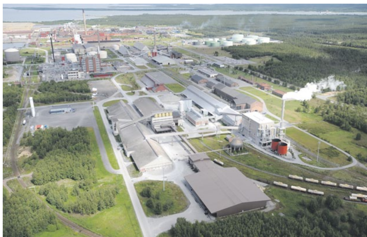
The Kokkola Industrial Park covers an area of 600 ha and therefore ranks among the ten biggest European Chemical Clusters.
