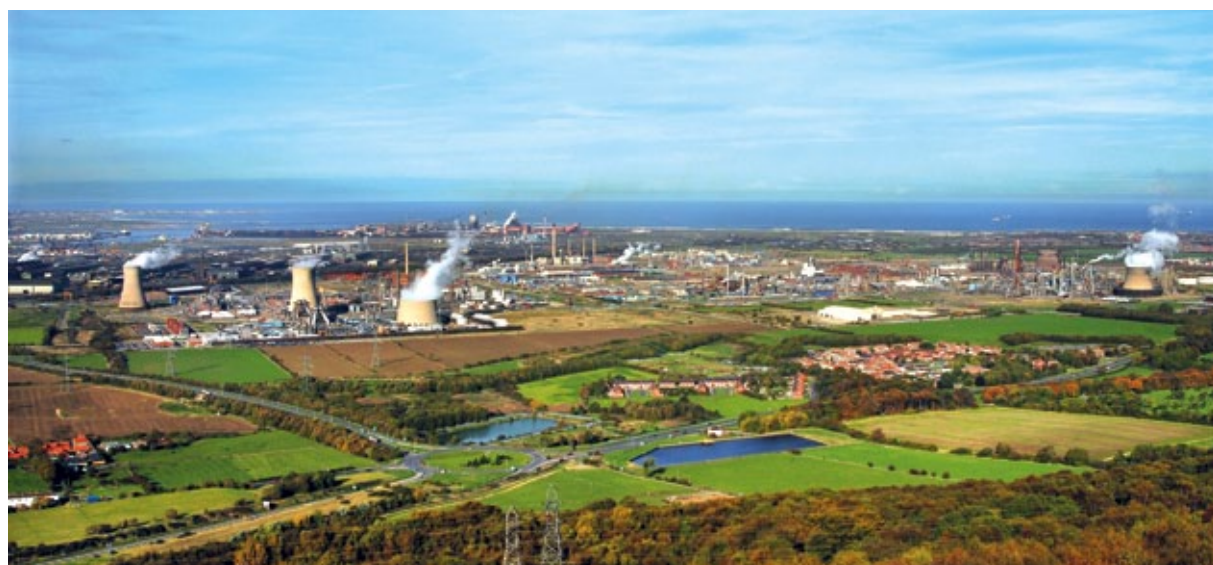
Wilton International chemical complex.
