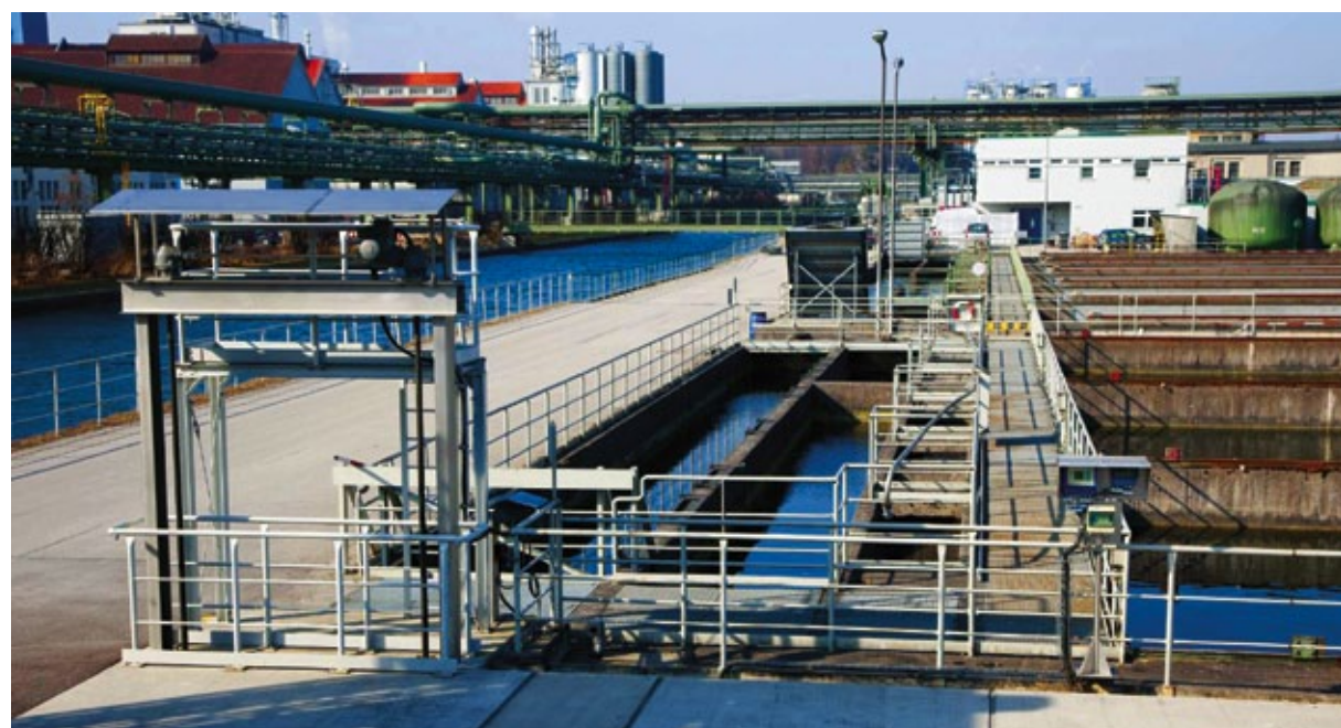
The Alz River, the Alz Canal and the sedimentation basins are — along with the Salzach and the Mühlbach rivers — important components of the cooling water supply system for all plant operations at Wacker Chemie in Burghausen.
