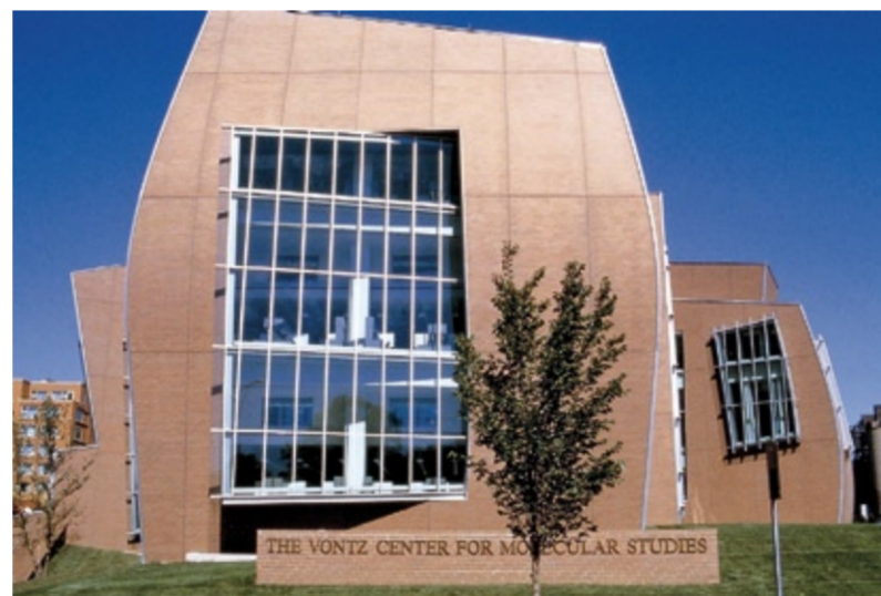
Modernity is also symbolized by the architecture: Frank O. Gehry designed the Vontz Center at the University of Cincinnati.
