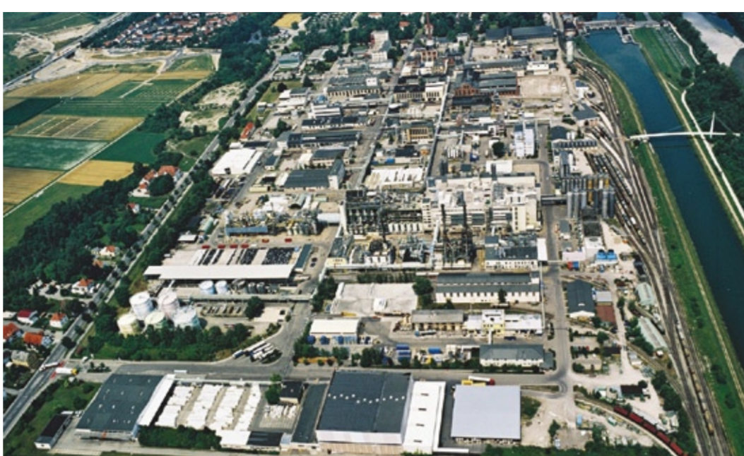
Fig. 1: At Gersthofen Industrial Park, approximately 1,650 employees work at 12 companies.
