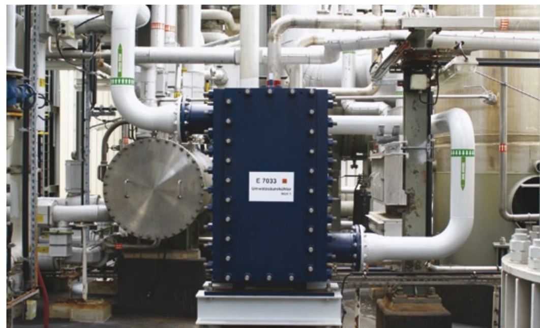
With a surface area of 54m 2 , over 200 plates and an output of 1,450 kW, the Gea Bloc keeps the hot nitric acid cool.
