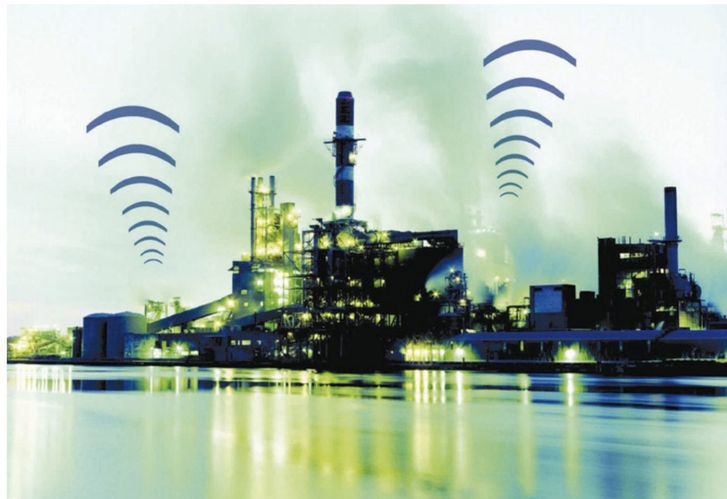
CAN YOU HEAR ME NOW? Typical environment for the use of wireless solutions in the process industry.
