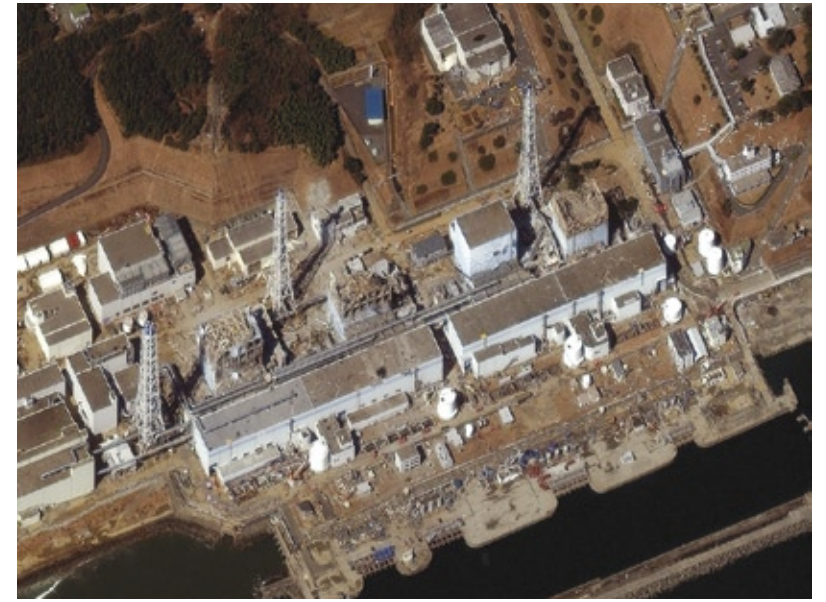
This satellite image of Fukushima Daiichi shows the remaining ruins of the plant. (Photo ©DigitalGlobe)
