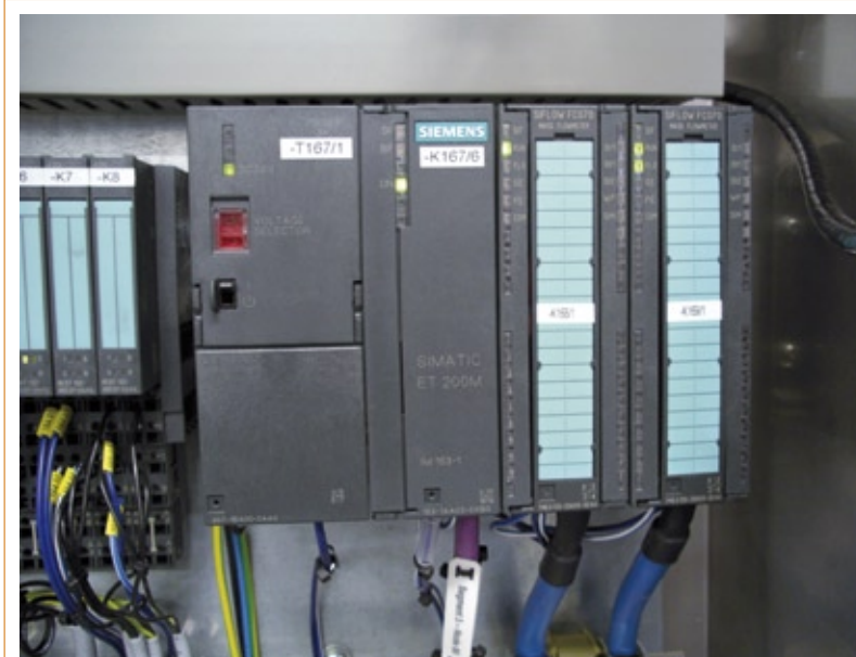
Siflow FC070 in the Simatic rack, fully integrated in the automation system over an ET200M Profibus node.
