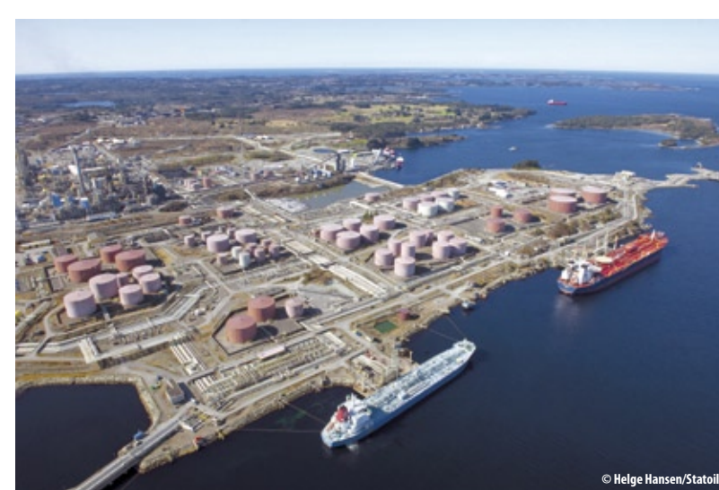
Mongstad oil refinery
